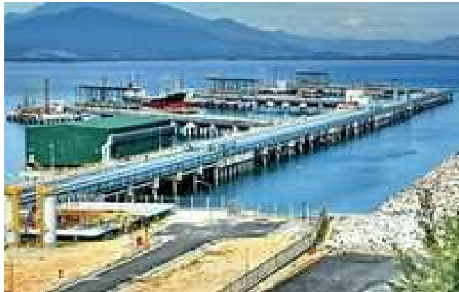
A seaport for exporting oil products at the Dung Quat Economic Zone in Quang Ngai Province
